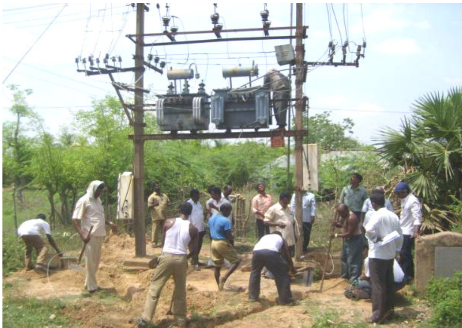
On Site Training to the Trainees
