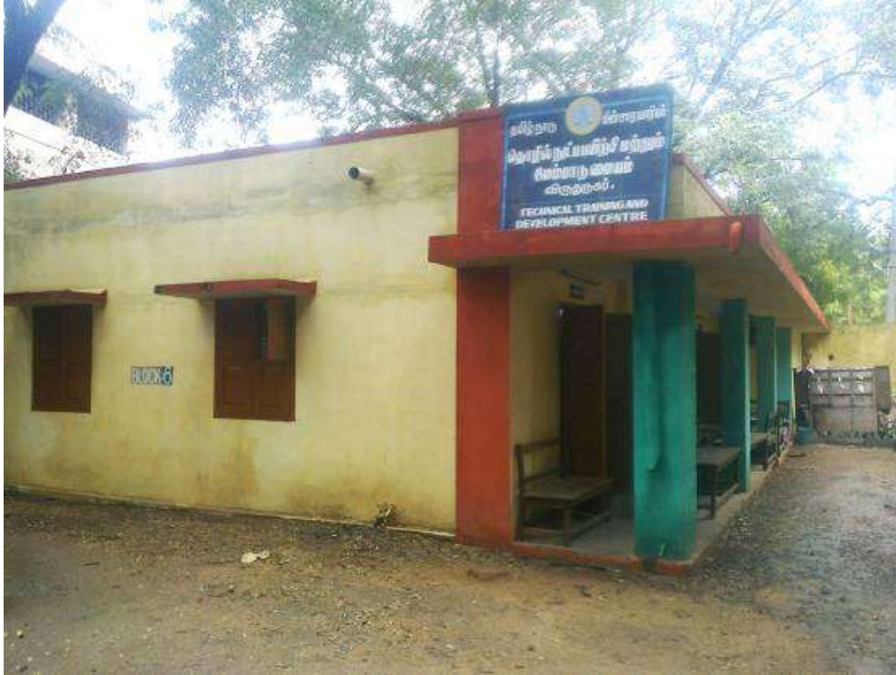
FRONT VIEW OF TECHNICAL TRAINING & DEVELOPMENT CENTRE , VIRUDHUNAGAR
