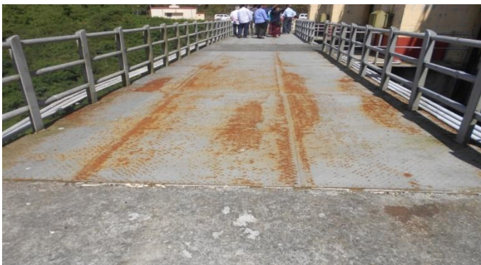
The rusting at spillway Deck Bridge
