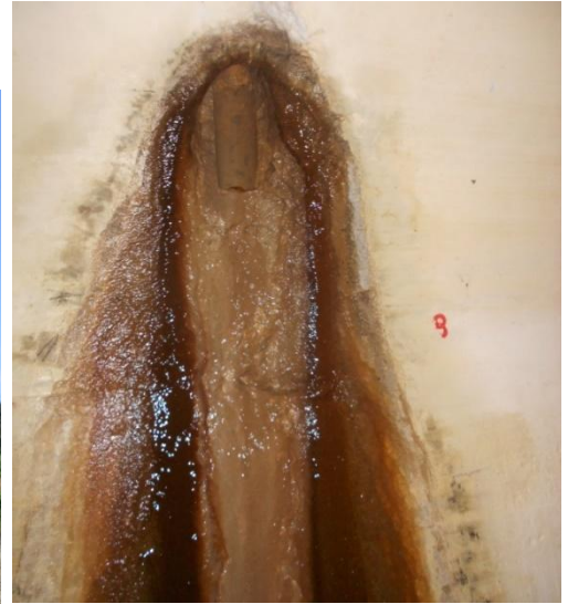
Calcination deposits from vertical shaft holes and gallery drain
