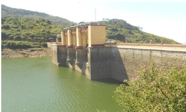
Upstream face treatment to be carried out to arrest the dam leaching
