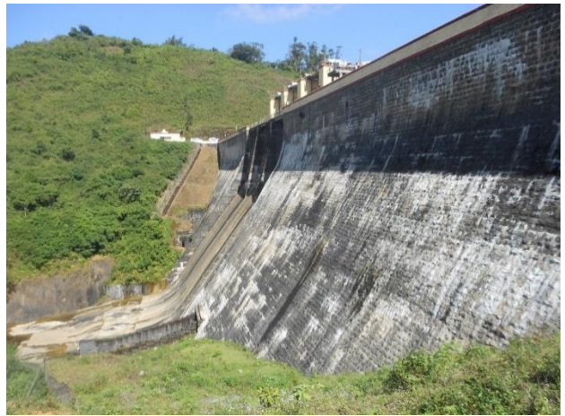
Downstream face of dam (leaching)
