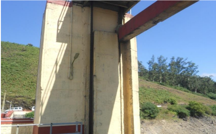
Exposed reinforcement of concrete counter weight
