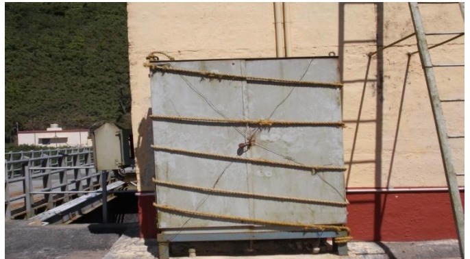
The damaged IT AC panel at dam top
