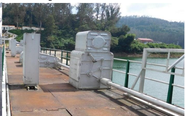
Chequered Plates at Hoisting Platform to be Replaced
