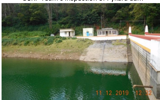
Masonry Dam Upstream Left Flank Protection Work
