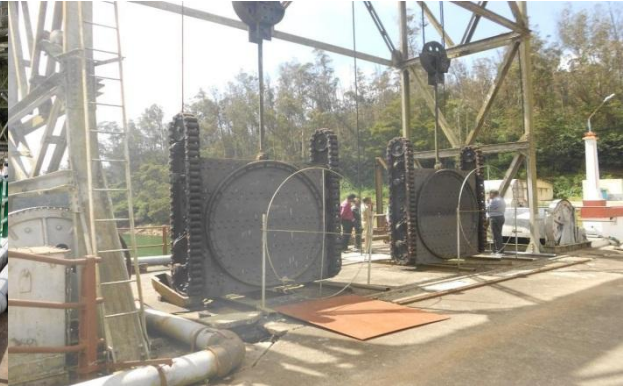
Overhauling of Scour vent Gate and Intake Gate to be Done
