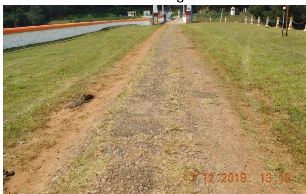
Earthen Dam top to be Concreted
