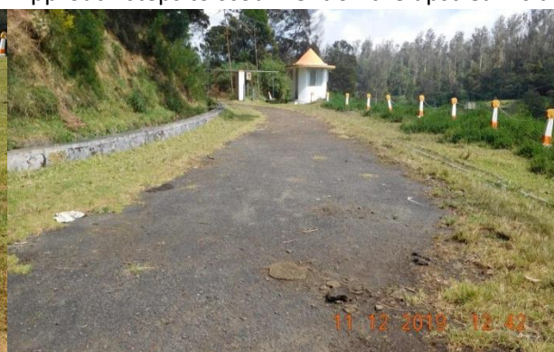
Approach road to dam on both Flanks to be Resurfaced
