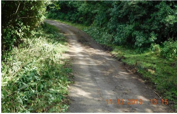
Approach road to Dam on both Flanks & Camp to be Resurfaced. ROW 3.50 m & Length 3.55 Km - there is no widening and tree cutting involved
