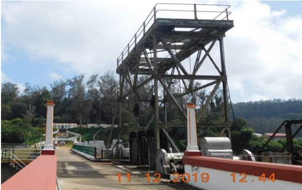
Extensive overhauling of Hoisting Mechanism and Replacement of Chequered Plates at Scour Vent Hoisting Platform to be Done
