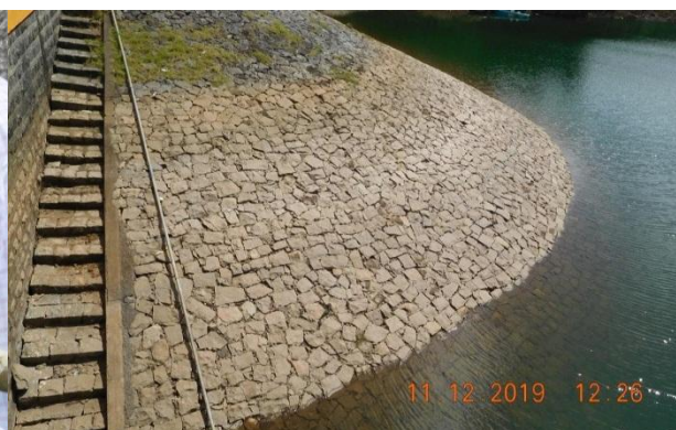
Earthen Dam Upstream Rip Rap
