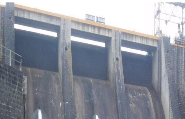
Overhauling, Welding and Painting of Spillway Gates to be Done
