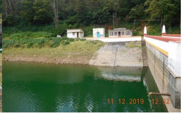
Upstream Left Flank Approach Steps to be Repaired
