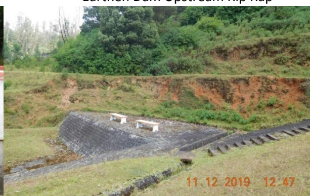
Downstream Right Flank Protection wall below catch water drain
