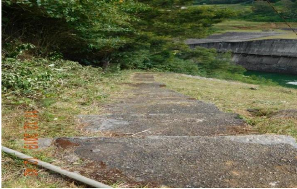
Left flank Down Streams Steps to be Repaired
