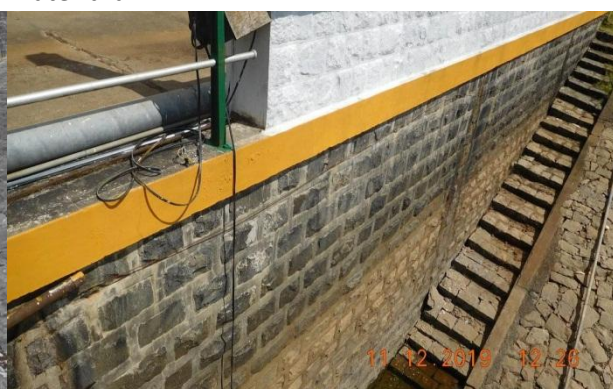
Approach steps to scour vent on the upstream side
